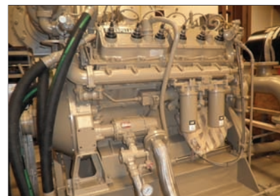
T106-F installed on Caterpillar 3412 engine.
